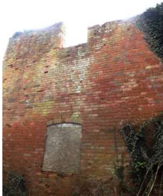
Figure 73 The mill building has now lost its upper two storeys
