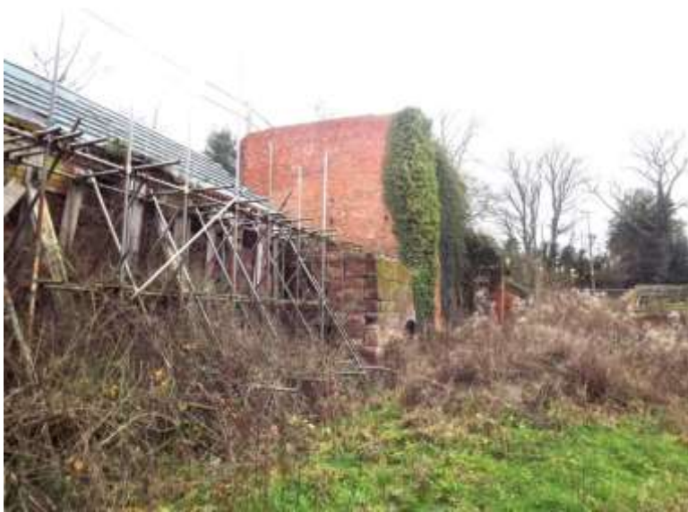
Figure 35 The grade II listed mill and maltings
