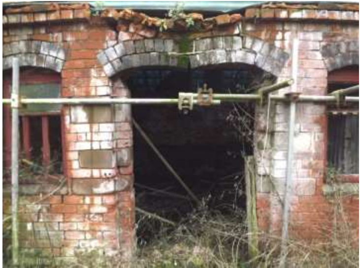
Figure 75 Wall collapse to the cart shed
