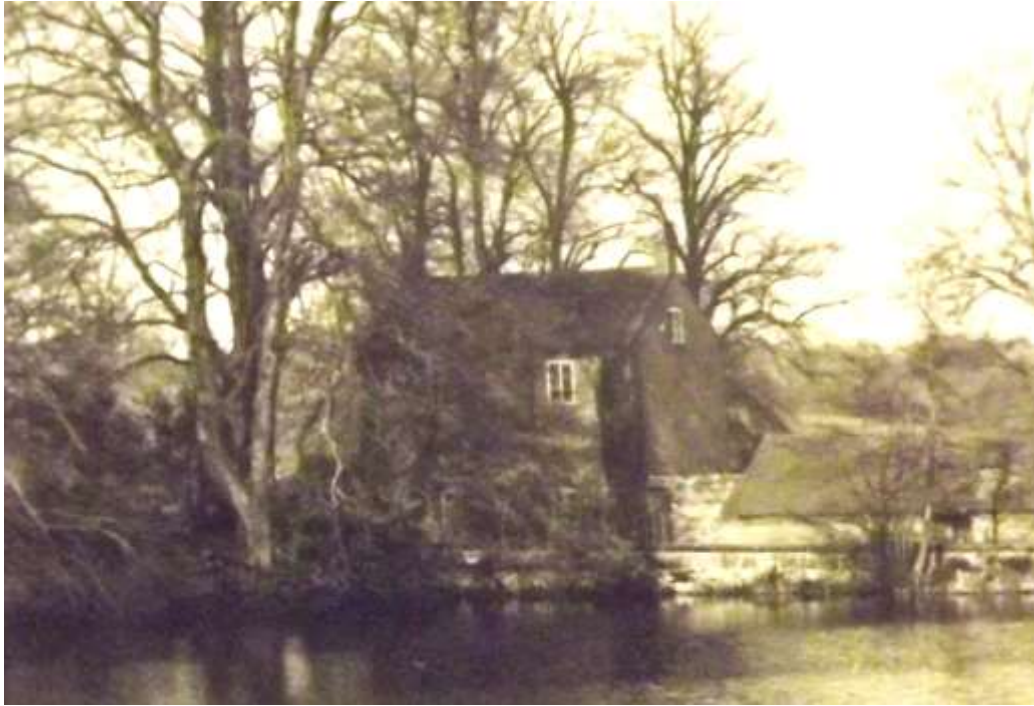
Figure 22 The front elevation of the mill c.1930, showing historic casement windows
