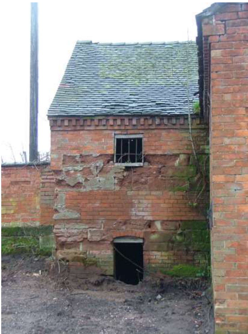
Figure 17 Courses of sandstone and brick to the maltings
