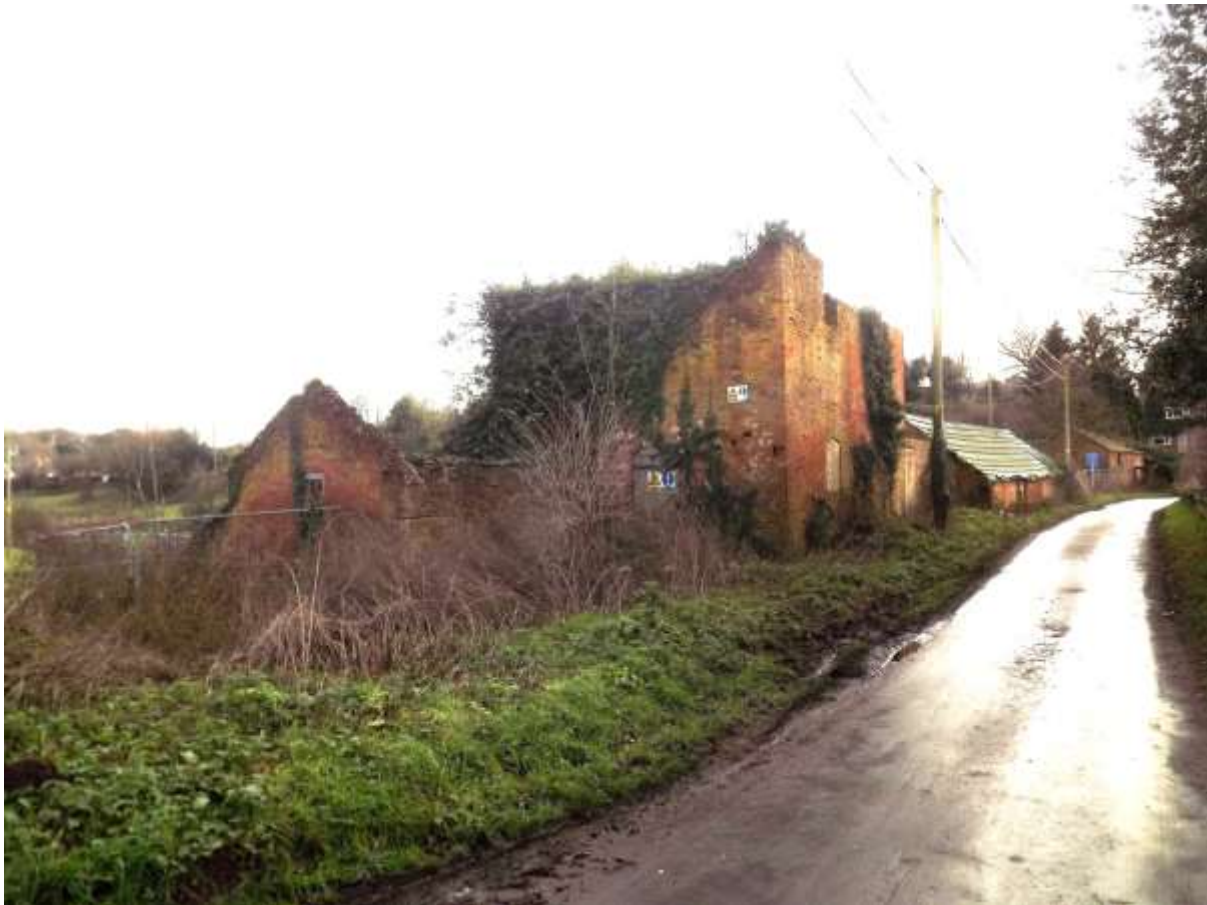
Figure 44 View of the mill and associated buildings from the north
