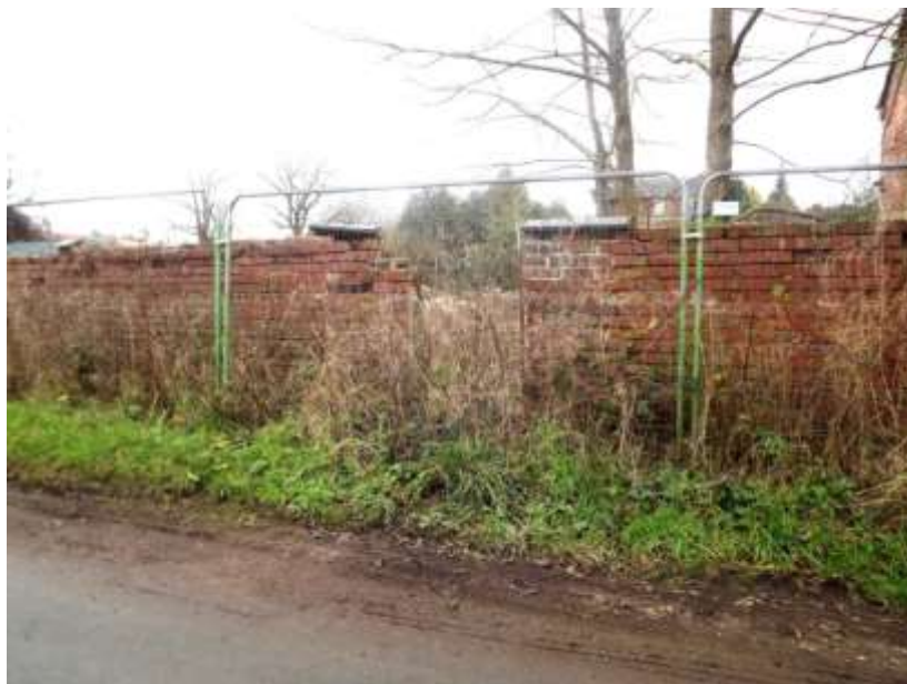
Figure 70 Brick boundary walls to the mill site
