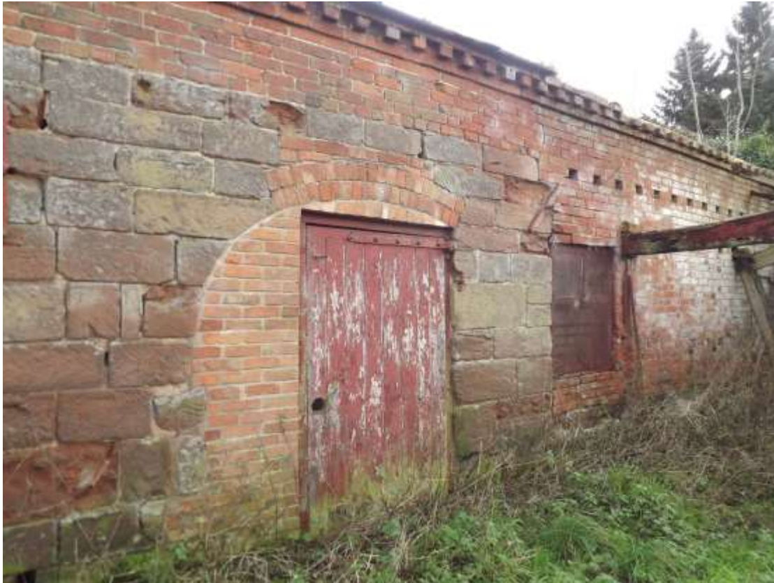
Figure 18 Combinations of sandstone and brick to front elevation of barn
