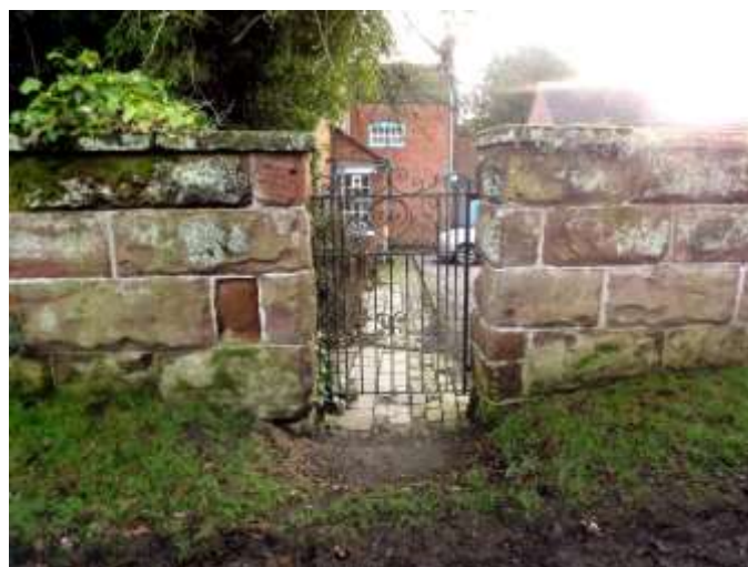
Figure 68 Stone walling and gate posts with historic metal gates to Walk Mill House
