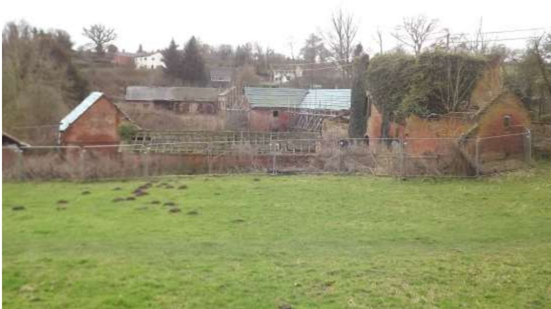
Figure 46 View of the mill from the public footpath
