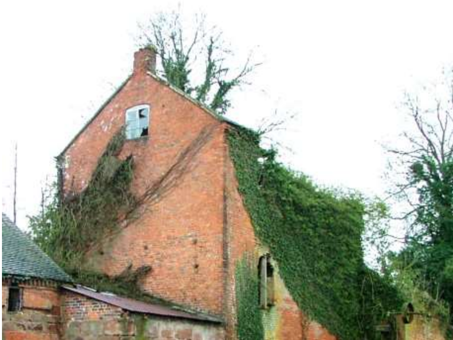
Figure 23 Side elevation of mill house c.2009, prior to loss of upper storeys, showing 3 pane side opening casement windows
