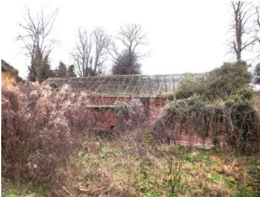
Figure 41 The piggery. Currently without roof tiles and in a dilapidated condition
