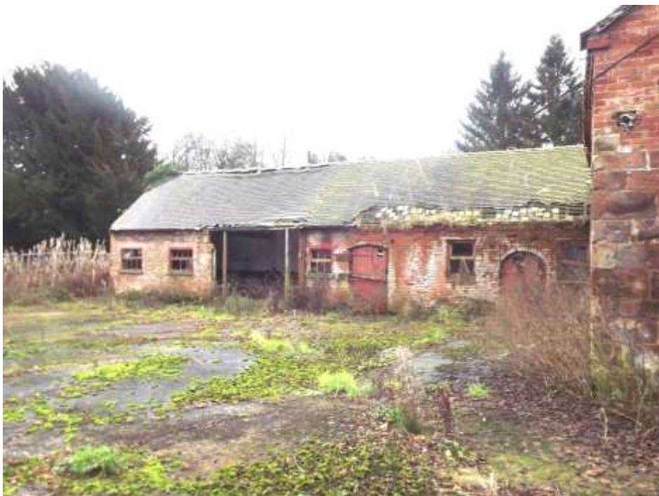
Figure 80 The cowshed to the rear of the former barn has been subject to heritage crime
