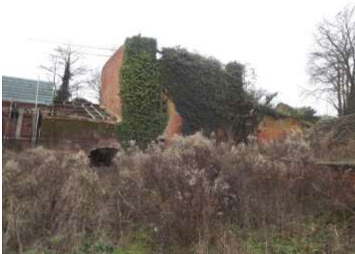
Figure 76 Excessive vegetation growth to the mill building
