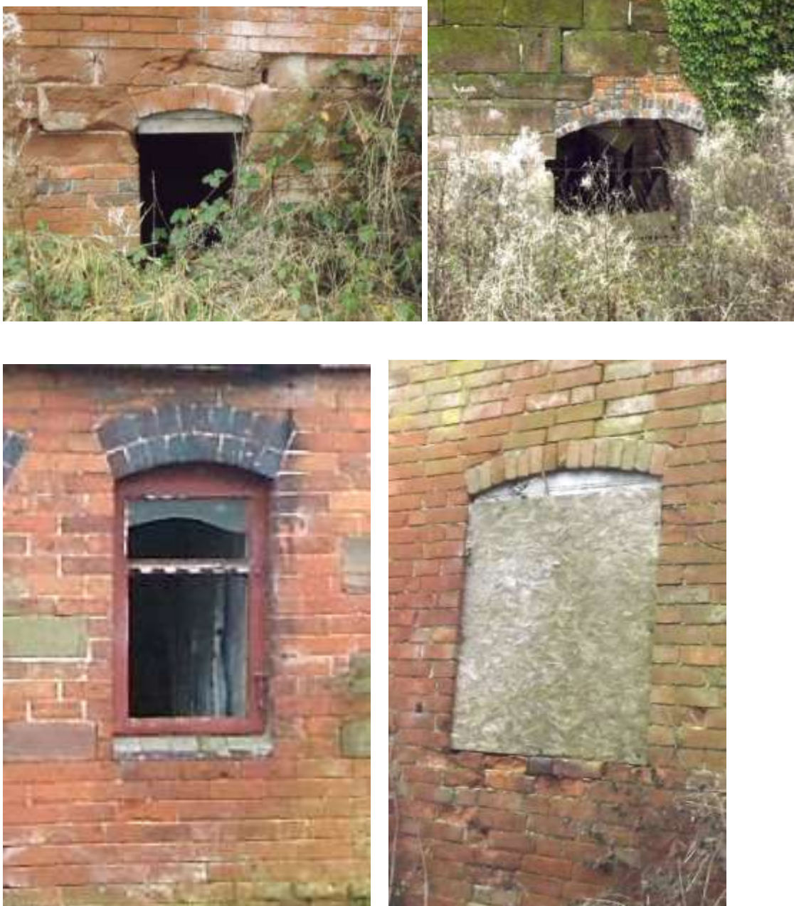
Figure 24 Variety of segmental arch lintels to windows
