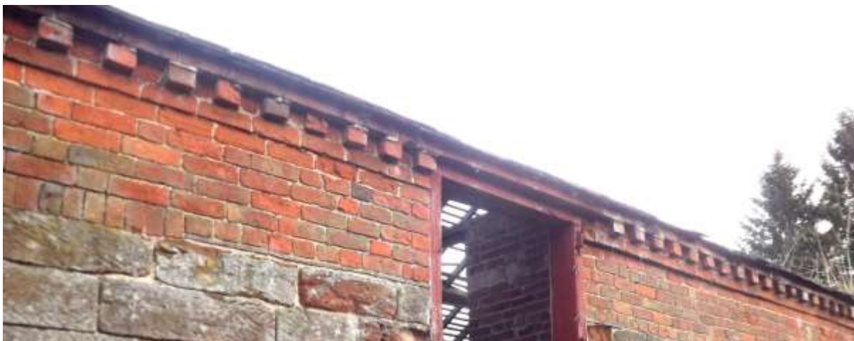
Figure 28 Dentilation to eaves to the maltings, Walk Mill Farm and the barn
