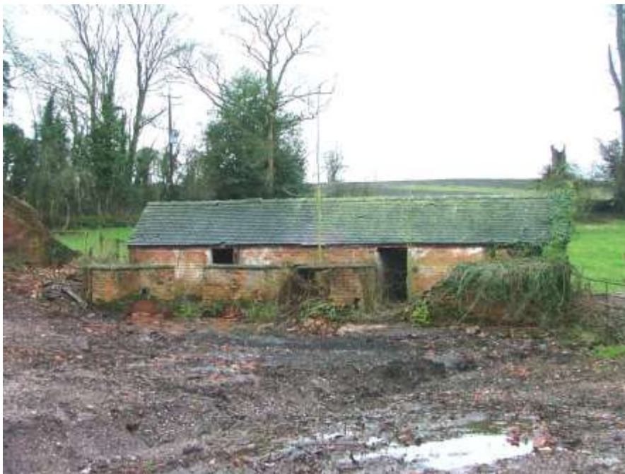
Figure 42 The piggery in 2009 prior to the removal of historic roof tiles.
