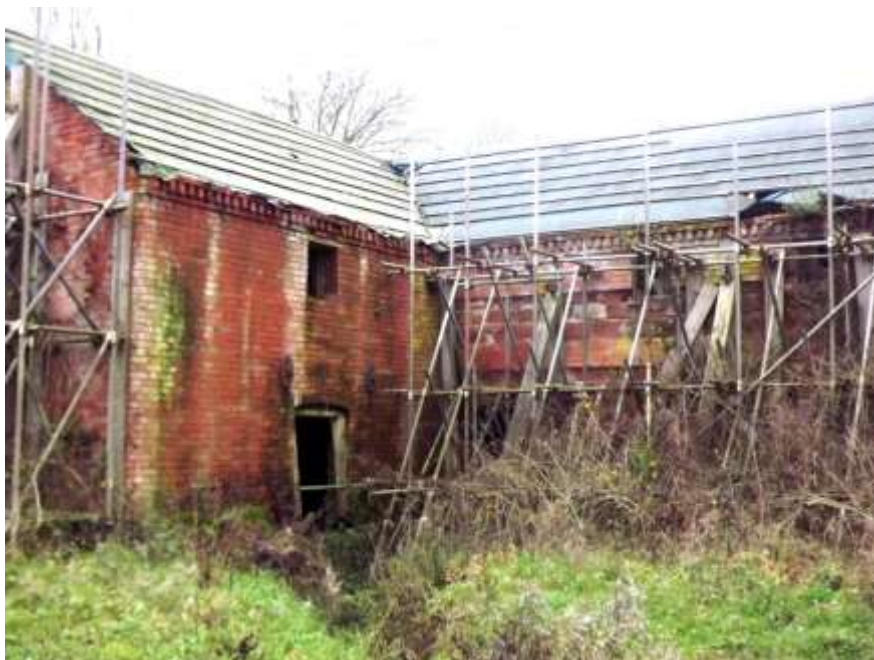
Figure 74 Scaffolding supports the former maltings
