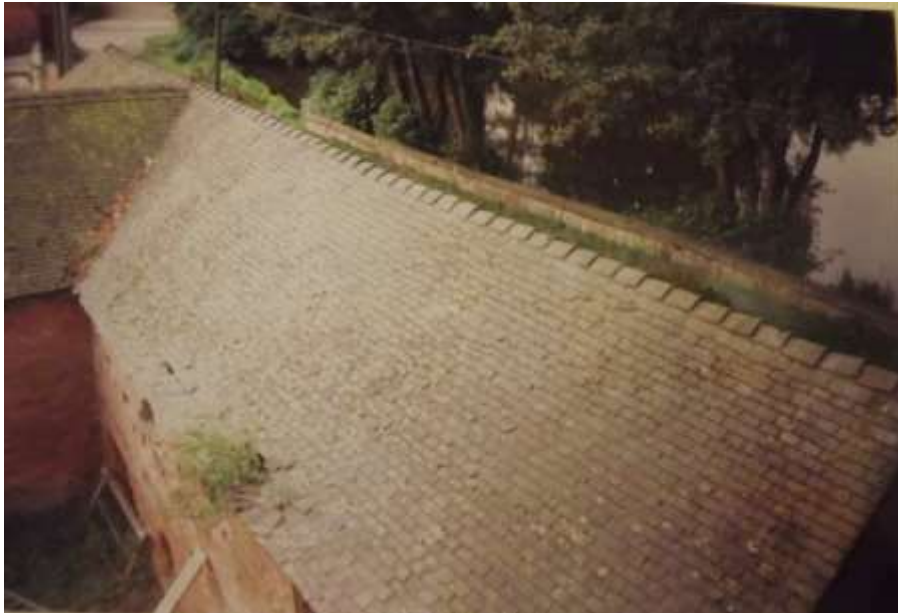
Figure 29 Staffordshire blue clay tiles to the roof of the maltings
