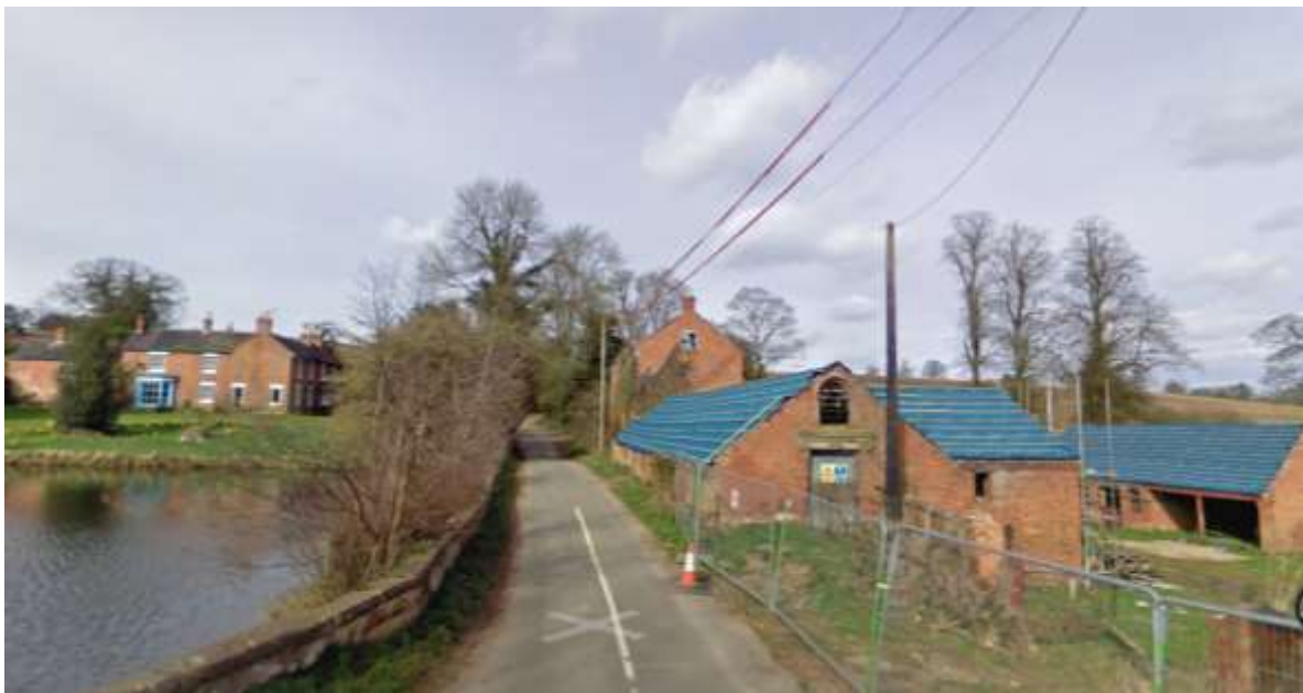
Figure 16 The three and a half storey mill building with top floors still intact shows the difference in scale and contrast to the lower storeyed maltings and agricultural buildings.
