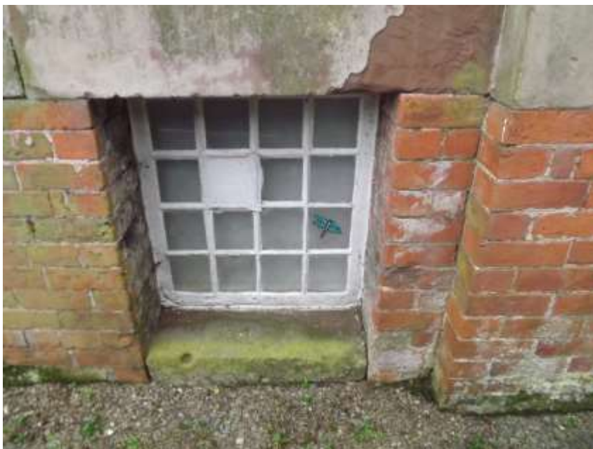
Figure 21 Cellar window to Walk Mill Farm
