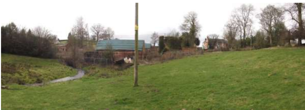
Figure 54 View of mill site looking west
