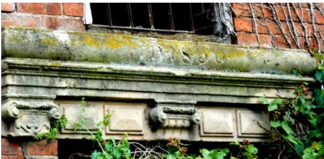
Figure 25 Moulded datestone lintel to maltings
