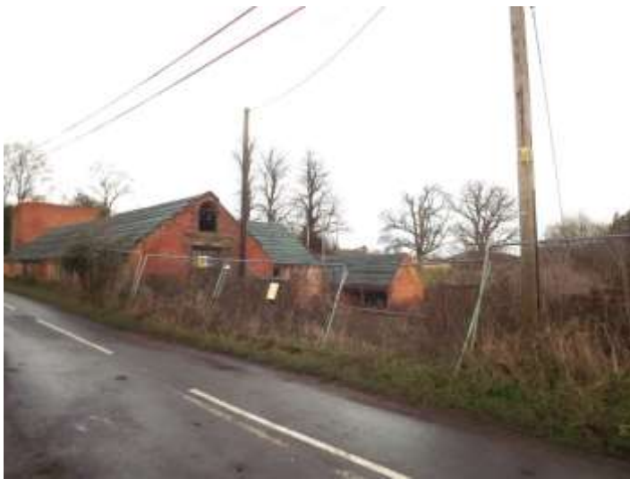
Figure 78 Weather proofing to roofs of mill and farm buildings
