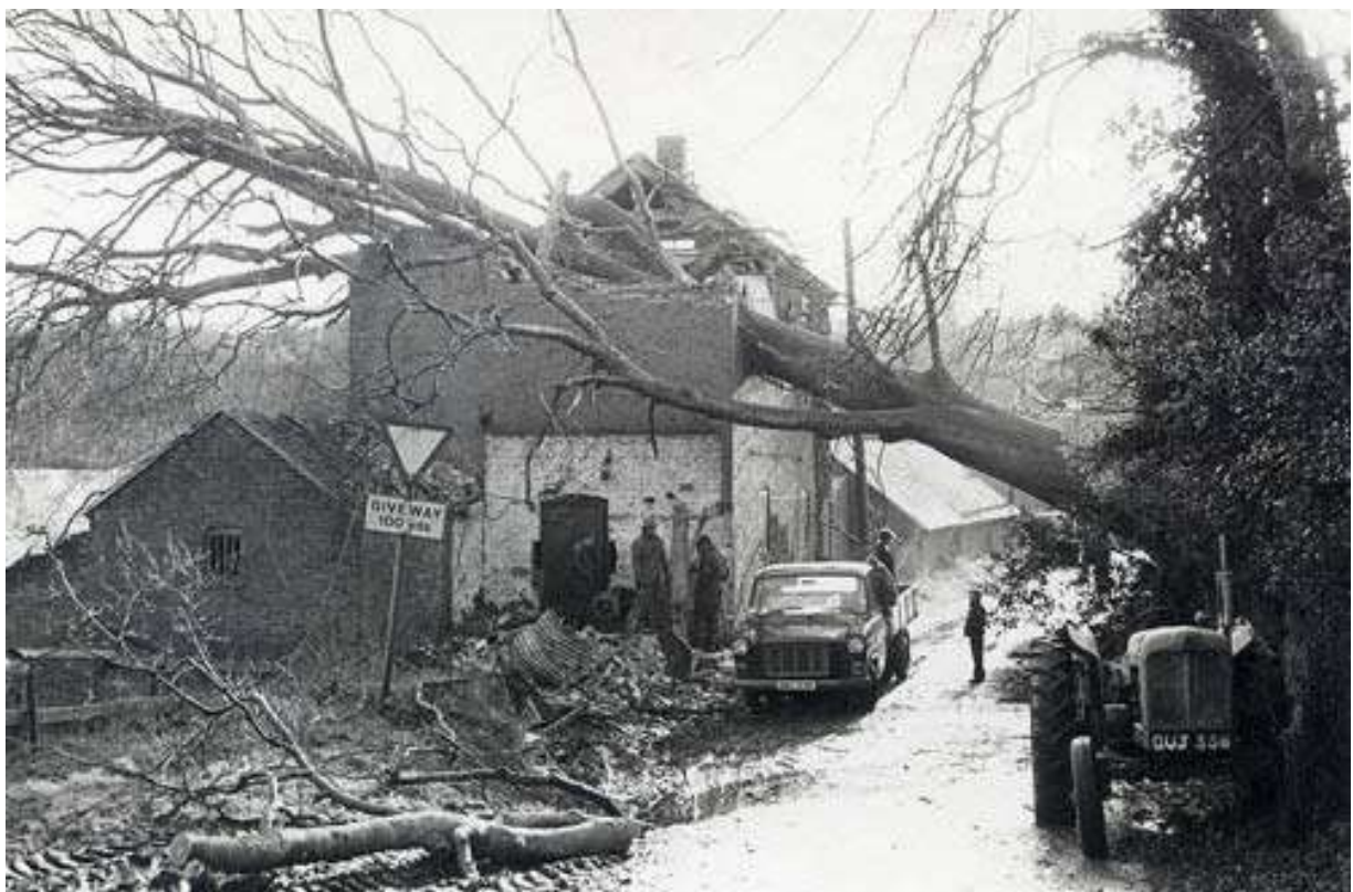
Figure 14 Storm damage to the mill in the 1970s
