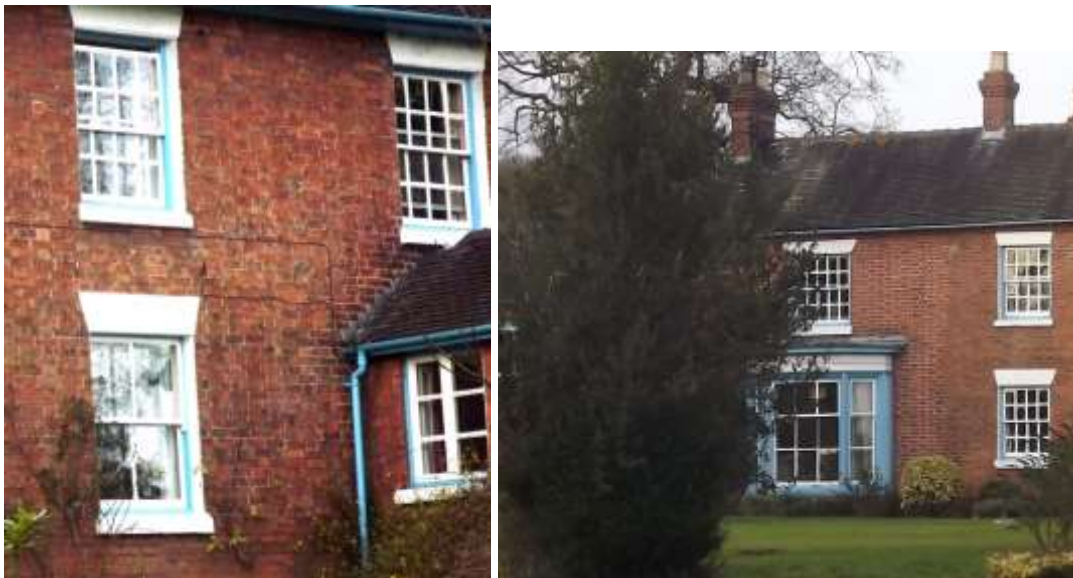
Figure 20 Sash windows to Walk Mill House
