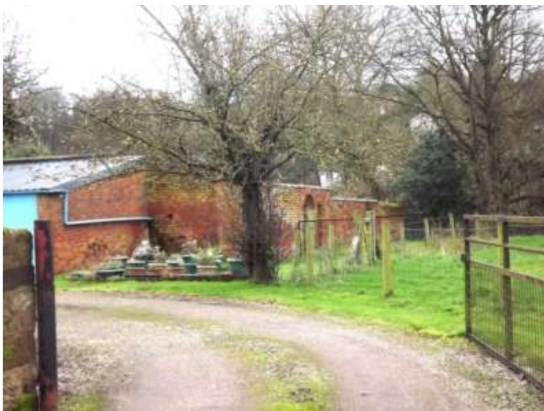
Figure 72 Walled garden wall in Walk Mill House grounds
