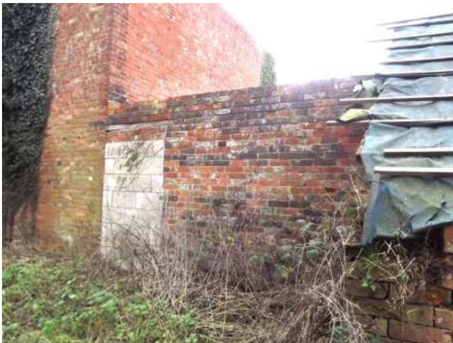
Figure 30 Blue and red brick to road side elevation of mill building
