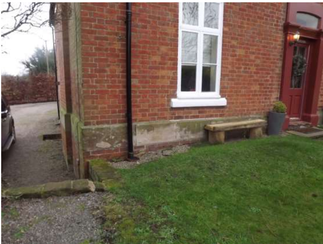
Figure 19 The use of brick and stone to Walk Mill Farmhouse
