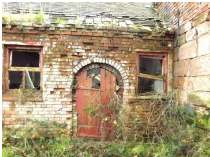
Figure 77 Damage and decay to cowshed
