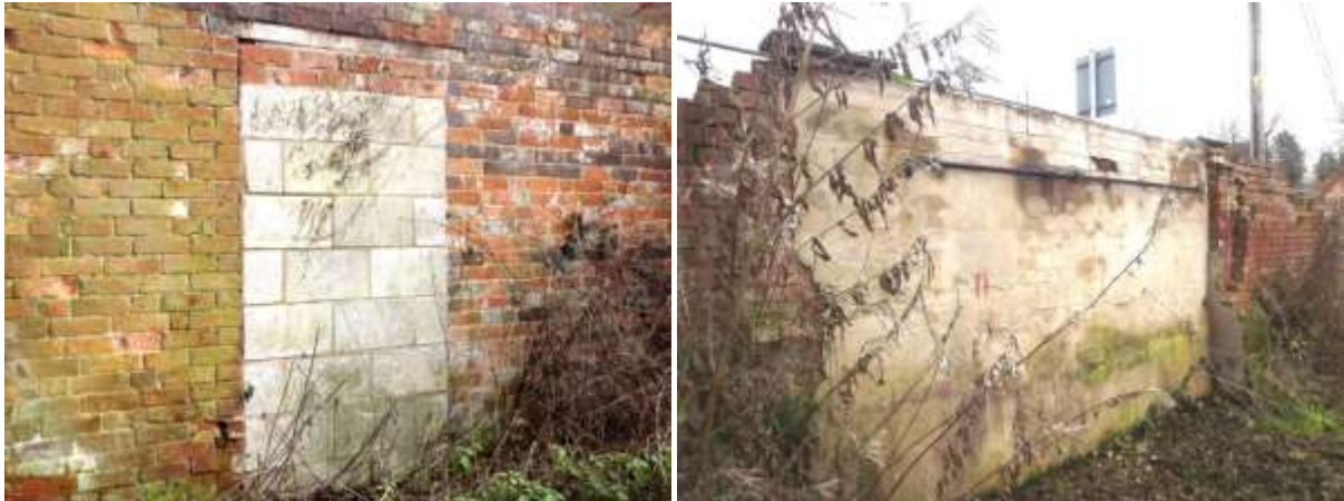
figure 79 Inappropriate materials used to block up doorways and cover walls have a negative impact on the Conservation Area.
